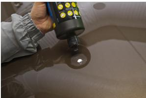
Apply one drop of Polarshine compound to the sanded surface.
